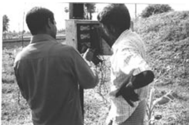
Photo-5: Measurement of Input power during technical evaluation in Erode, Tamil Nadu
